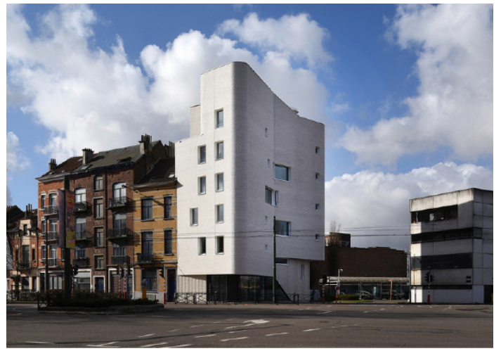
REF: Navez House, V+ & MSA, Schaerbeek
